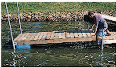
Lift and remove sections
