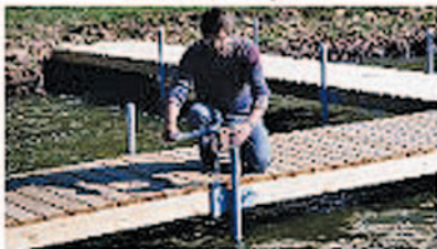
Use winch to lift pipes
