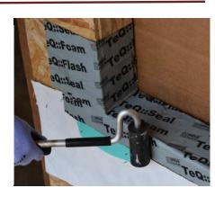
Recommended Sealant: QuadMax™ by Henkel/OSI®, Recommended Flashing Tape: TiteSeal™ Butyl Self Adhering Flashing; Butyl Flash, by OSI/Henkel.
