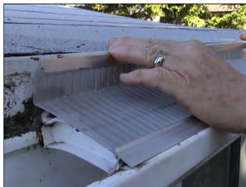
Bending mesh to fit small gutters.
