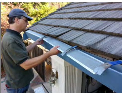
Flat bars used to lift up tile.
