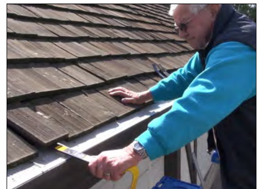
Using flat bars to lift up wood shake.
