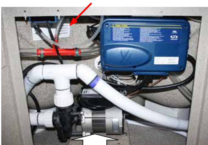
110 Volt Equipment Compartment
