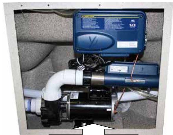
230 Volt Equipment Compartment
