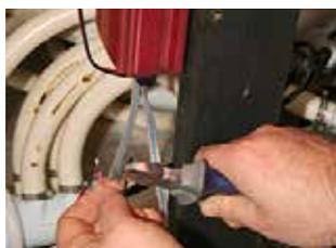
**STEP 8** - Remove insulation cover from wires.
