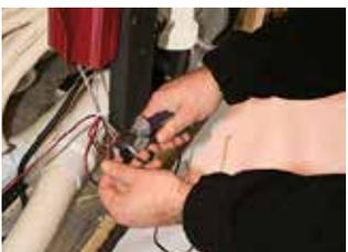
**STEP 5** - Cut Black/Red and Red wires on amplifier wires.
