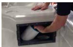
**Step 4.** Replace with the new filter(s) and rescrew filter(s)
