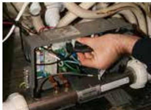
**STEP 6** - Remove clamp to wire - unplug pump plug from circuit board (ensure cable ties are removed from plumbing)
