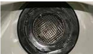
**Step 1.** Removing the basket and filter can be done with or without water in the spa/hot tub (Tip: when lifting filter from water have a net or sieve in hand to catch any residual dirt).
