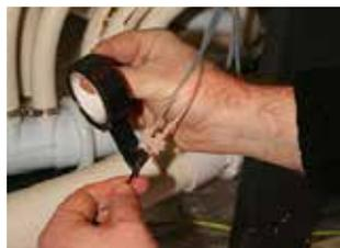
**STEP 7** - Insulate tape wires and block before reassembly
