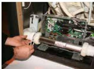
**STEP 9** - Remove gaskets from plumbing and fit new ones from new heater
