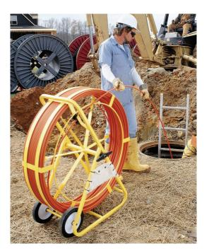
Heavy duty non-conductive rodder for manhole-to-manhole work or long-run cable pulls. With the ability to operate vertically or horizontally, the Big Buddy® has the versatility to handle the toughest jobs.
