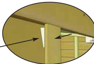
**31.** Locate 2 **Door Trim Spacers (4D)** found in the Hardware Bag with **Plywood Spacer (UU)**. Slide door spacer between door trim and wall siding. Attach with 1 -  $1 1/2''$  **Finishing Nail (K)**. Nail through trim and into spacer. **Complete attachment of door trim using 4 more  $1 1/2''$  Finishing Nails (K).** Make sure to align trim accordingly. Complete both sides.
