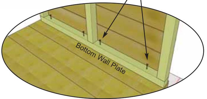
6. Starting with angled left side wall, lift up and position so framing is flush with floor at rear of shed. Make sure wall siding is flush with outside of floor on the side. In the front, there will be a gap of approximately 5/8". When wall is positioned correctly, secure bottom wall plate to floor with **4 - 2 1/2" Screws (C)**.
