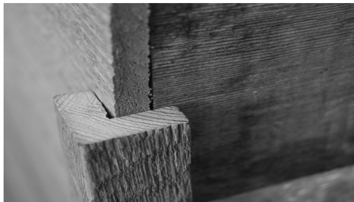
Figure B - If you are stopping on the flat wall leave a 1/2" space and cover the edges with our flat wall trim pieces.
