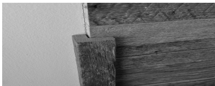
Figure C - Depending on the board width, apply adhesive as in and place the first row on lightly.
