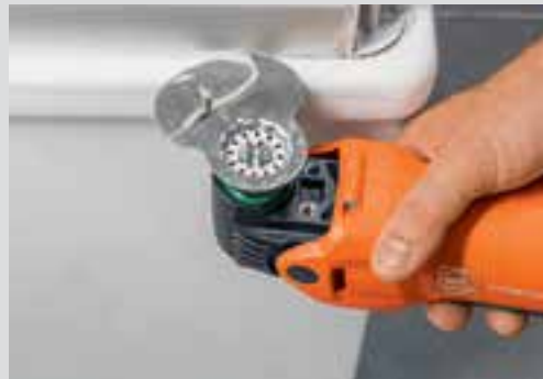
Remove connection joints.
