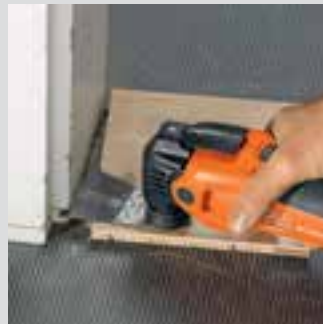
Work flush with the surface.
