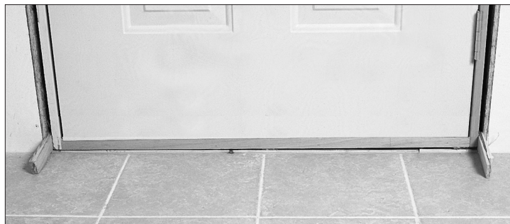
Figure 13: Proper position of shims at the bottom of the door (Points A).
