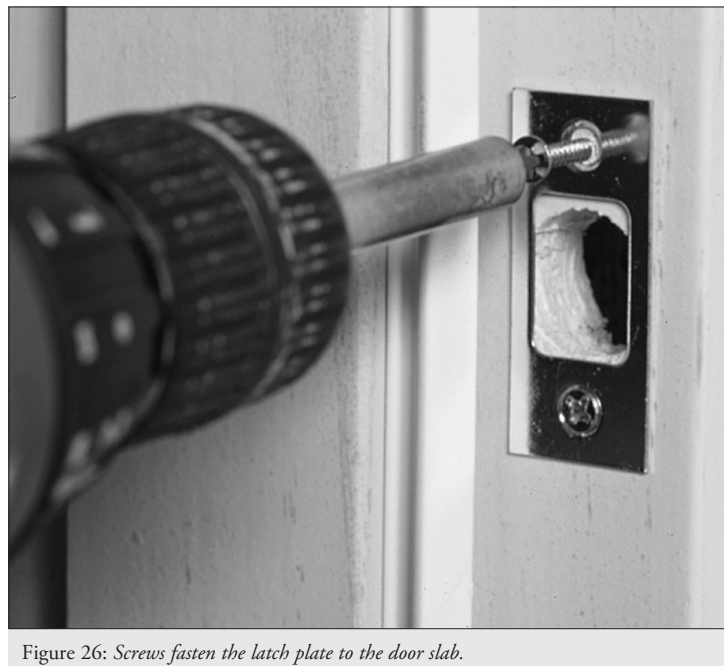
Figure 26: Screws fasten the latch plate to the door slab.
