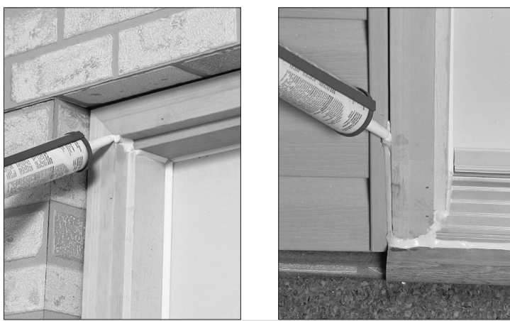
Figures 30 and 31: Caulk the jambs and the exterior trim.
