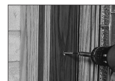
Figure 25: Drill holes through the exterior jamb on factory-finished jamba and fill in holes with fill stick provided in hardware bag.
