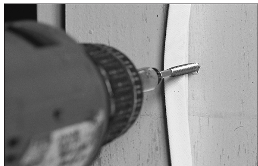
Figure 15: Install screws underneath the weather-stripping. It is strongly recommended that you remove the weather-stripping to ensure that you do not pierce or puncture it.
