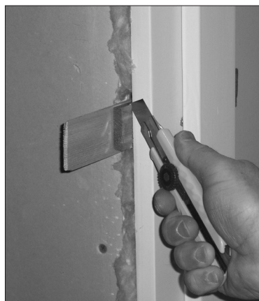
Figure 27: Insulate between the jambs and the wall studs all around the door.
