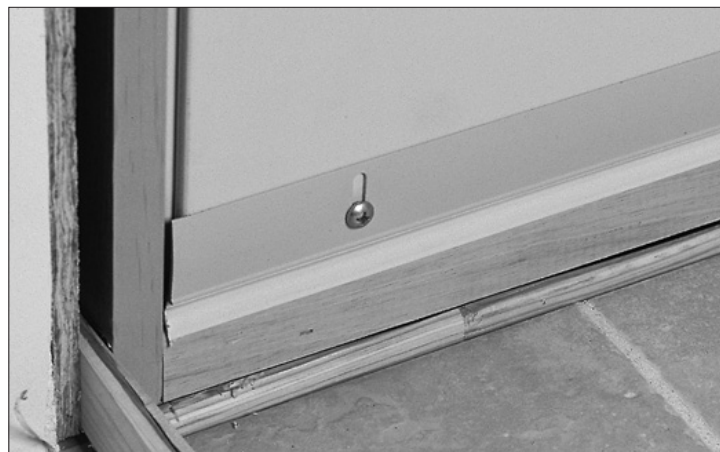
Figure 33: U-channel sweeps are adjusted to form a tight seal with the sill.
