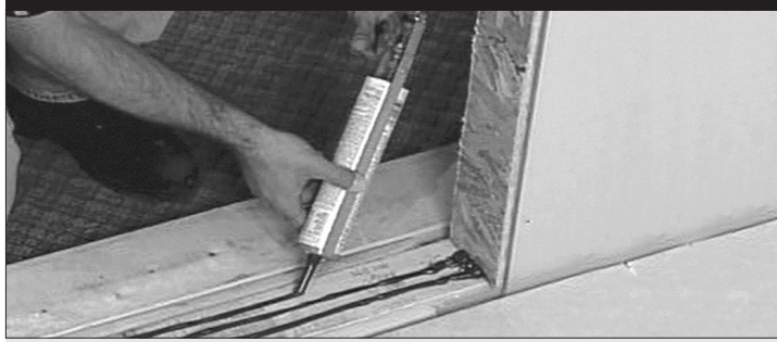
Figure 2: Caulk is applied in three parallel lines running the width of the sill.
