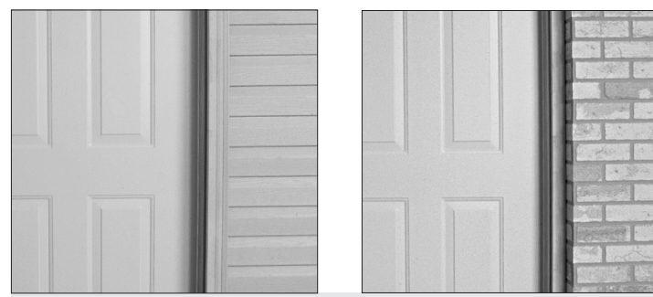
Figures 7 and 8: The exterior trim (brickmould) rests up against exterior sheathing or slides into the opening of exterior brick.
