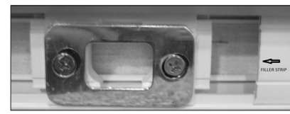
Figure 20: Aluminum Astragal Strike Plate adjustment.
