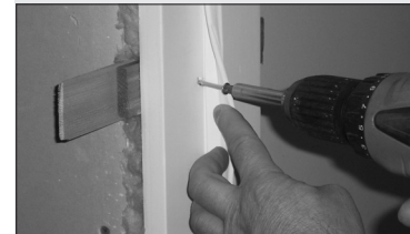
Figure 11: Screws are installed through the jamb, shims and into the 2x wood studs or backing. It is strongly recommended that you remove the weather-stripping to ensure that you do not pierce or puncture it.
