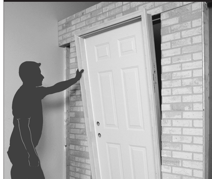
Figure 6: Place the sill in the opening first and then tilt the door up into the opening.
