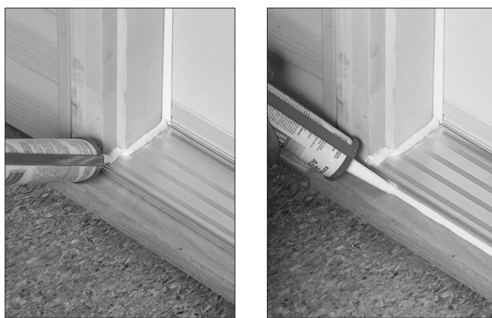
Figures 28 and 29: Caulk the sill crown and the front of the sill.
