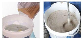
Mix using an electric drill with the paddle at low speed until achieving a smooth mixture without lumps. When the 2 components are properly mixed you will notice a homogeneous, uniform paste without color variation. Scrape the sides and bottom of the bucket with a spatula or trowel to ensure complete and proper mixing. It is never advisable to mix by hand.
