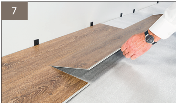
Figure 7: Continue alternating planks on rows 1 and 2. Insure planks are properly aligned along the chalk line and against the spacers. Finish rows 1 and 2 in this manner, cutting planks at the end of the row as necessary. Insure that the end planks are a minimum of 6" in length. If necessary, adjust the length of starter pieces to insure minimum plank lengths for each row, with proper end joint stagger row to row.
