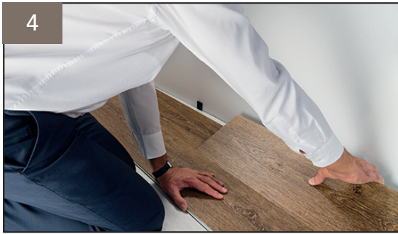
Figure 4: Working from the wall, insert plank 3 into the long side of plank 2.
