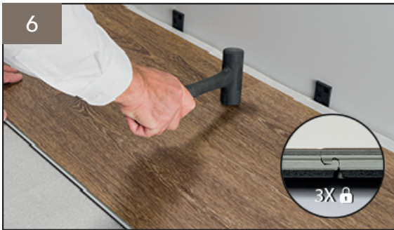
Figure 6: Using a rubber mallet, lightly tap the joint on the short side to engage the locking system.
