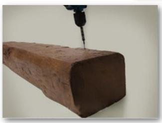
3. Then put screws through the top of the mantel to anchor it into the 2 x 4. You could apply construction adhesive on the edge of the mantel for extra security.
