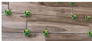
Large format Tile floor Install
