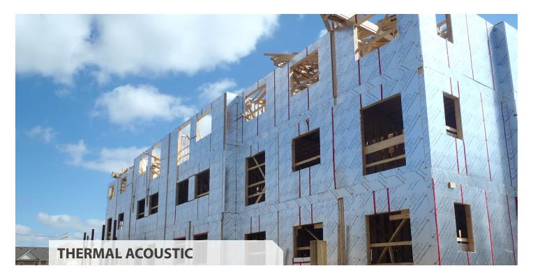
SilveRboard Acoustic is a Do-It-Yourself (DIY) nonstructural, rigid insulation board made from closed cell Expanded Polystyrene (EPS) with a layer of reflective metalized polypropylene film laminated on both sides.
