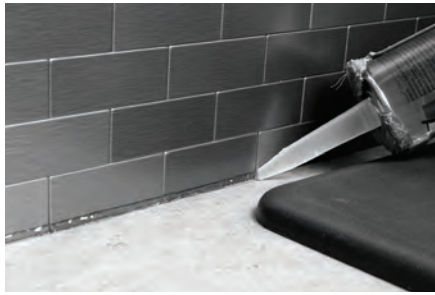
Caulking the counter top seam
