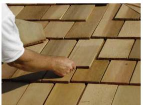
**50.** Slide in another Filler Shingle and attach as per **Step 49.** On your last row of shingles, the filler shingle is precut to fit properly. Attach to roof with 2 finishing nails per shingle.
