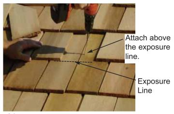
**49.** Screw first filler shingle down to rafters using 1 - 2 1/2" screw per panel (2 in total). Make sure to screw into both rafters.
