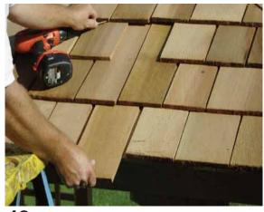
**48.** Roof **Filler Shingles** are included to cover roof seams. Starting at the bottom, slide the first Long Filler Shingle in until flush with other bottom shingles. **See step 49 for proper attachment.**
