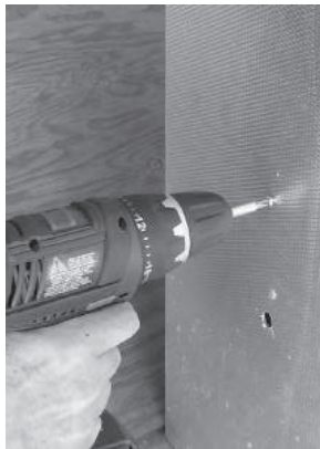
Install Hanger Screw
