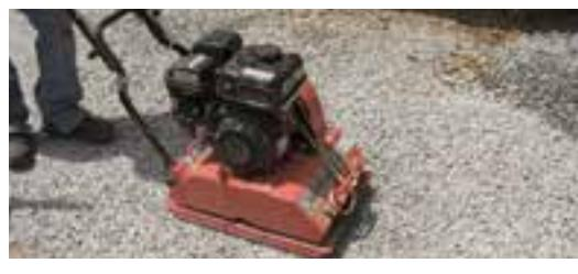
Prepare a sub-base to a depth of 4" using  $\frac{3}{4}$ " crushed gravel to allow for drainage and stability. Compact the sub base and level off, ensuring a 2% slope away from any buildings or foundations. Gently mist the compacted sub base to further compact this layer.
