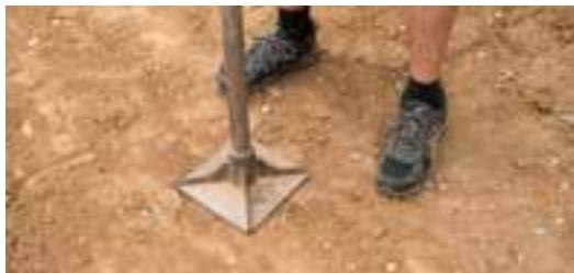
Compact the soil ensuring a minimum of 2% slope away from buildings and foundations. This will increase the load bearing strength of the soil, and minimize movement due to freezing or thawing and other seasonal changes.
