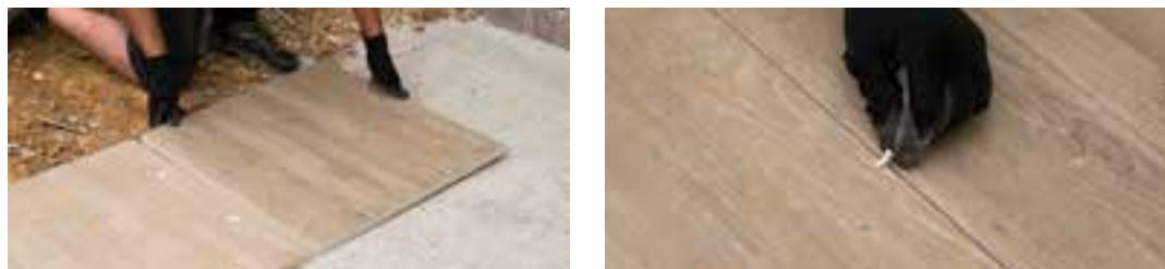
Select size and color of the pavers and place them gently on the prepared surface. Complete the laying scheme according to the project specifications or to your preferences.
