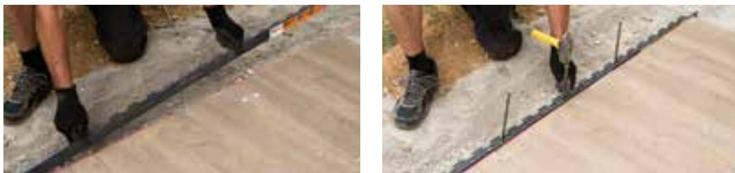
Install edge restraints according to project specifications, and the indications of the restraint producer. This will help reduce horizontal creeping, and the loss paver base at the edges of the installation. Edge restraints should be tall enough to contain paver base material and pavers, but not higher than the installation ( $1 \frac{3}{4}$ "). The edge restrain will be installed on top of the landscape fabric and will be instrumental in containing the paver base material and the pavers.
