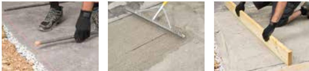
Lay 1" thick pipe (screed rails) parallel every couple of feet. Fill with 1" of paver base material. Pass a flat board over the screed rails to level out paver base, ensuring a slope of at least 2% away from any buildings or foundations. Remove screed rails and fill gaps with paver base material, and smooth the newly filled in gaps.
