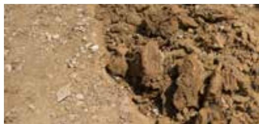
When digging make sure to dig a depth that will include the entire base. The depth of the base will be determined by preexisting soil and climate conditions in your area. Most normal soils will require a total depth of 5"
