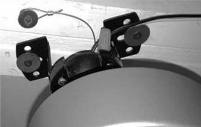
Photo 5: Safety cable attached near hanger
