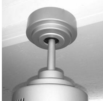
Photo 6: Complete hanger assembly
