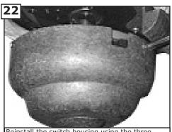
Reinstall the switch housing using the three screws previously removed.
