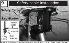
For Canadian installation and for USA fan and light kit combinations over 35 lbs, in both flush and downrod modes the safety cable must be installed into the house structure beams using 3" lag screws, washers and lock washers provided. Make sure that when the safety cable is fully extended the lead wires are longer than the cable and no stress is placed on the lead wires. **Note**:If Installing The Secondary Support Safety Cable in the U.S., Do Not Remove Knockouts In The Outlet
