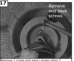
Remove 1 screw and save.Loosen other 2 screws.
