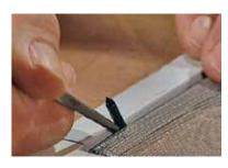
spline material being pried up from the sliding door frame before old screen removal
