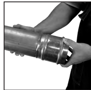
Figure 9: Inspection of final crimp
