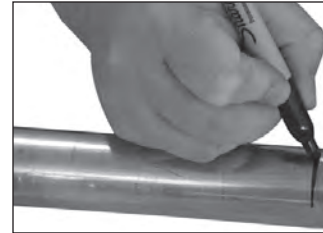
Figure 3 — Marking for Insertion Depth
