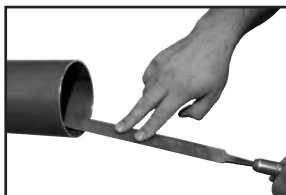
Figure 2: Deburr inside diameter using a half-round file
