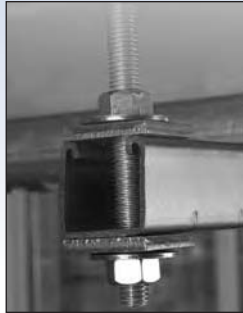
Standard method using nuts and washers.
