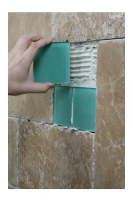
joint placement guidelines in EJ171 in the TCNA Handbook should be followed. Movement joints should be placed every eight feet with a caulk meeting the requirements of ASTM C920. Custom Building Products Commercial 100% Silicone Caulk meets this requirement.
