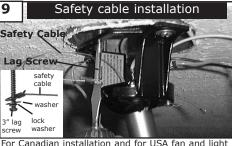
For Canadian installation and for USA fan and light kit combinations over 35 lbs, in both flush and downrod modes the safety cable must be installed into the house structure beams using 3" lag screws, washers and lock washers provided. Make sure that when the safety cable is fully extended the lead wires are longer than the cable and no stress is placed on the lead wires. **Note**:If Installing The Secondary Support Safety Cable in the U.S., Do Not Remove Knockouts In The Outlet Box.
