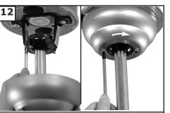
Loosen one and remove one pre-assembled screw from mounting bracket. Save screw. Lift canopy up, aligning its keyhole slot with the pre-assembled screw on mounting bracket and twist clockwise to lock in place. Re-install the removed screw and tighten all screws securely.
