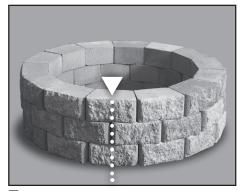
**7**. After the 2nd layer is finished, install the 3rd by placing the center of each block in line with the joint of the blocks below. When the 3rd course is all lined up, glue the blocks one-at-a-time as in step 6.
