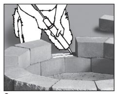
**6.** Once the 2nd course is all lined up, carefully remove one block at a time and apply two thick beads of concrete adhesive to the center of the blocks. Reinstall the block and push down firmly. Continue for all remaining blocks on 2nd course.
