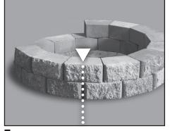
**5.** After the 1st course is set and leveled. start the 2nd course by placing the center of the top block in alignment with the joint between the blocks below. Continue this all the way around the circle.
