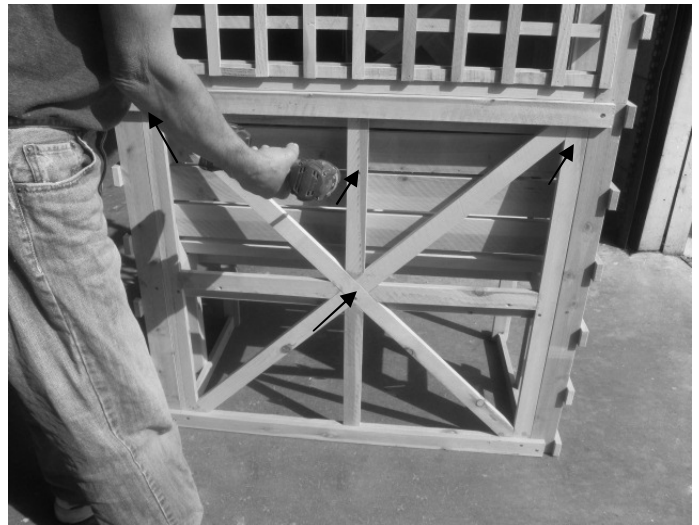
16. Fasten the back frame and bench with screws.
