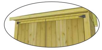
**62.** Place **Above Door Trim** on door header between door trims. Attach with 6 - 1 1/2" nails. Leave small gap to allow for proper door opening and closing.
