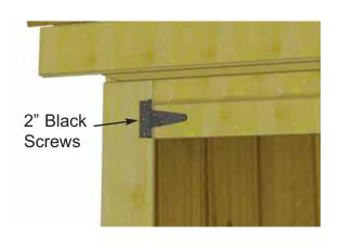
**60.** With Door correctly aligned, attach Door Hinge to Door Trim with 2" black screws. **Hint:** Do not attach all the 2" screws in each hinge until both doors are positioned correctly into place. Drill pilot holes in Door Trim prevent wood from splitting. When satisfied with door positioning, complete all 2" screws then.
