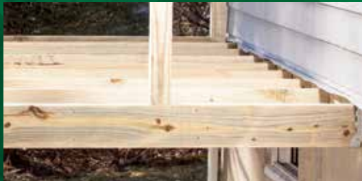
Deck Ledger Attachment
