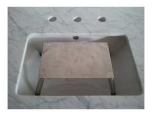
3. Adjust all 4 legs, one leg at a time by twisting it, so the stand's top surface is at the same level/surface of the bottom of the stone top surface as shown.
