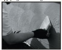
back to texture it before the coating begins to dry. Adding up to 12 ounces of water per 5 gallon pail of TUFF II will make it easier to work with while texturing. Remember to try to work to natural stops, like inside and
