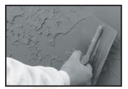
brush texture, use a large nylon bristled brush kept moist in a pail of clean water. A knockdown texture can be achieved by stippling the TUFF II with a trowel and then knocking it down. Continue moving along the wall, applying the coating to an area and then quickly going
