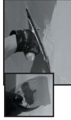
Sticky Mesh HD is sold in rolls 150 feet long in 9.5", 19" and 38" widths. The Sticky Mesh adds strength to the wall and helps bridge seams and gaps. Overlap runs of mesh by two inches.
