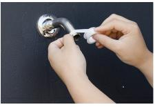
Apply the included Teflon tape by wrapping it around the shower arm threads a few times.
