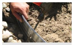
6 Drive spikes through holes in edging at a 45 degree angle. Start with the beginning piece of edging.
