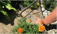
**5** Cut edging section to the desired length at the end of the bed area using a hacksaw.
