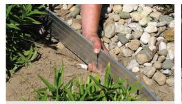
Slide ends of edging strips together to connect pieces. Adjacent section of edging can be connected prior to or after the sections are in place. Overlap: minimum 2"; preferred: 4".
