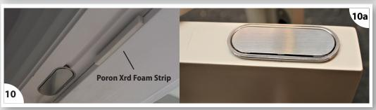
10. Once the desired magnetic holding strength has been achieved, affix the **SELF ADHESIVE S/STEEL COVERPLATES** to the magnetic face(s) of the ASSEMBLIES as shown, to protect the magnets from corrosion and for a more attractive 'concealed fix' finish. (10, 10a)
