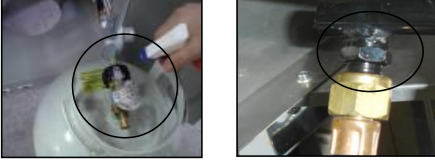
Gas Connection Leak Check
