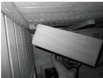
FIG 15.2 Installing the Radio Wood Housing
