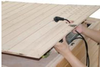
FIG 17 Slip the power cord through Roof Cover
