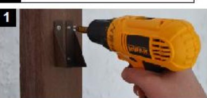
1 Attach Brackets : Use chart to find rail heights. Measure up from ground, mark post for bracket bottom. Attach with provided screws. Secure rails into brackets with screws.
