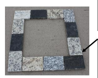
**Step 1**:Level the pad. Level an area of gravel or rock on compacted soil that is approximately 40" X 40" for the 21" Square Fire Pit Kit or 49" X 49" for the 30" Fire Pit Kit. The leveling pad will be approximately 6" larger than the fire pit kit.
