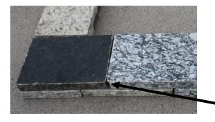
**Step 3**: Install second course of blocks. Place a block on top of the bottom corner block staggering the intersection of two blocks on the course below. Continue around the fire pit making slight adjustments as needed so that the edge of the blocks fit together. When the 2<sup>nd</sup> course is in place, remove the blocks one at a time and adhere each block to the blocks below using quarter sized dabs of a quality construction adhesive.
