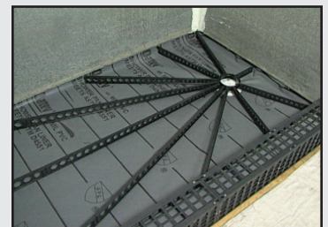
Quick-Pitch® Standard and Extended and Kirb-Perfect® installed.
