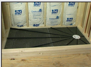
Positionnement brut des extensions Pre-Pitch MC et Pre-Pitch MC standards.
