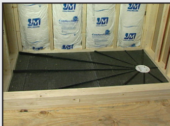
Pre-Pitch™ Standard and Extended installed in rough-in.
