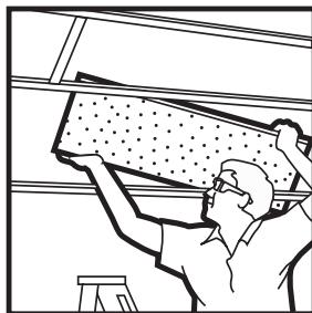
**12. Lay in the ceiling panels** — It's easiest to begin in one corner of the room and install panels one row at a time. Tilt each panel up through the opening and lower it to rest squarely on all four tees. Note: Arrows on panel backs should all point in the same direction!
