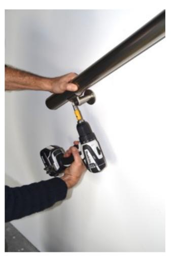
Screw the pipe onto the wall mounts using the included screws
