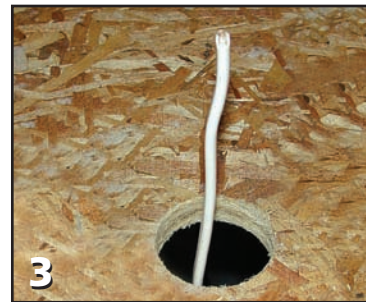
Figure 3 - Pull Romex wire through floor.
