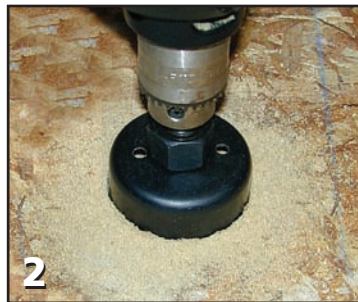
Figure 2 - Drill hole in floor using a hole saw.
