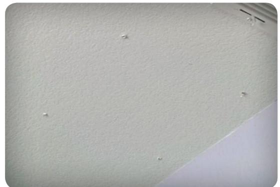
3. From below, place the cut-out template on the ceiling, making sure that you have at least 2 inches of clearance all around it. While holding the template in place, mark its outline with a pencil.
