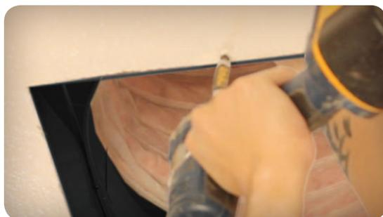
10. Remove ceiling grille and screws from its packaging. Center the grille over the damper box. Install the grille with the white screws provided by screwing through the drywall into the flange of the damper box.
