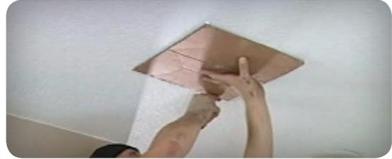
4. Using a drywall saw or similar device, cut out the hole in the ceiling.
