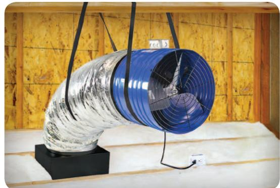
7. Hang the motor head from the rafters by fastening the metal strapping that is attached to the motor heads to the rafters with the wood screws. Make sure that the handy box on the motor head is at the very top. Secure duct to damper box using three black sharp screws. Make sure the housing is angled slightly up and the duct has a gentle 90 degree bend to help reduce noise level. The angle is important so the fan does not disturb any blown-in insulation in your attic.
