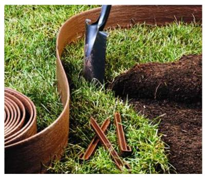
Use a rope or garden hose to lay out a line where you plan to install the edging. Trench approximately 4 In. to 5 In. depending on the type of edging and desired appearance.
