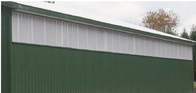
Eavelights economically allow natural lighting into the building. Eavelights are made of Polycarbonate and are available in soft white. Polycarbonate is extremely weather resistant, will not yellow in harsh sun, and is recyclable. Panels come in 36” widths.
