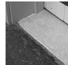
ASPHALT TO CONCRETE
