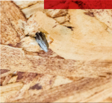
Roofing nails piercing roof decking
