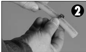
2 Slide clamp or crimp ring over tube.
