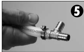
5 Verify connection is secure. Use go/no-go gauge on crimp rings.
