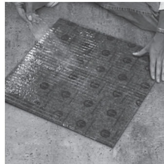
Remove peel-off backing and slide carpet tile into position on the floor.
